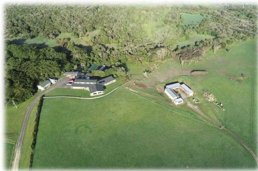
Henga Lodge and Marakapia Lookout featuring new roof
